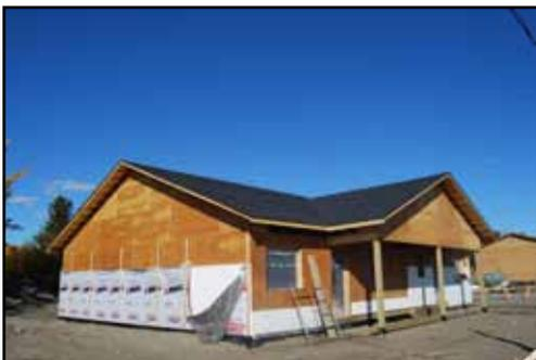
As many Citizens will know a home was previously built on this site that had to be moved. The cause was an uncapped well, underneath the foundations that went undetected. After the home was built the well lead to the basement being flooded which continuously rendered the property uninhabitable. The well has now been capped, the new duplex has no basement which was part of the problem, and proper drainage has been installed.
