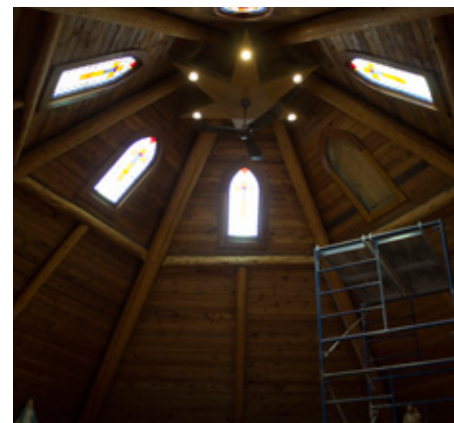
Catholic Church windows- The church was built in 1970 and the stained glass windows have started to rot and leak. The framing will be replaced to hold the stained glass windows securely.
